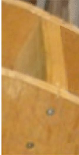
Personally, I would like the screws to be offset so that neither is on the centre line of the plank as that is the weakest arrangement, and so I suggest that the two screws are positioned one third of the way in from the plank edge as that gives a stronger connection with the screws 13 mm apart and not stressing the timber along one plane.
